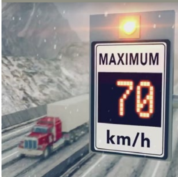
Exhibit 3: Variable speed limit sign
