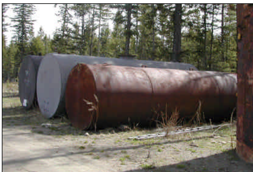
Faulty storage stanks can leak contaminants into surrounding soil
