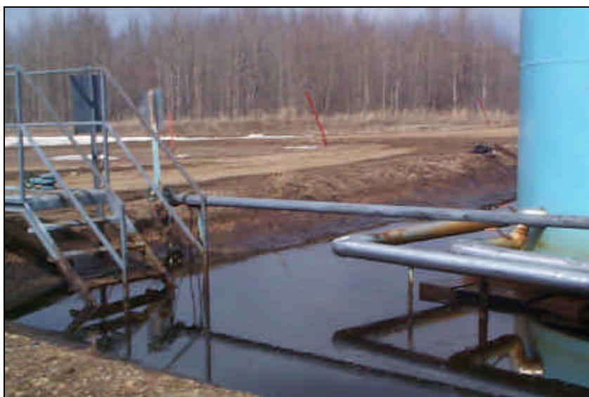
Berm containing leaked oil
