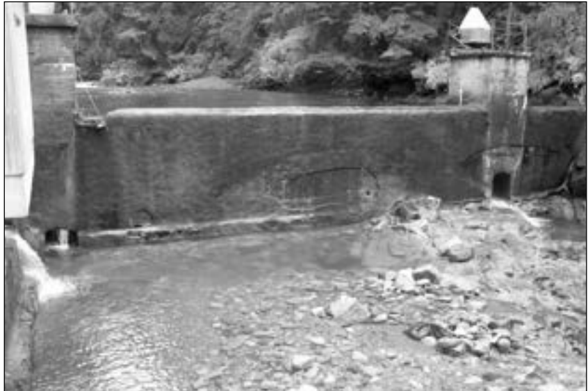
Water impoundment obstructing fish passage
